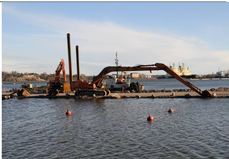
Figure 94 A dredger at work in near Helsinki, Finland. (Photo: Metsähallitus)
