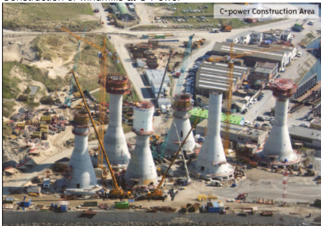
Construction of windmills at C-Power
