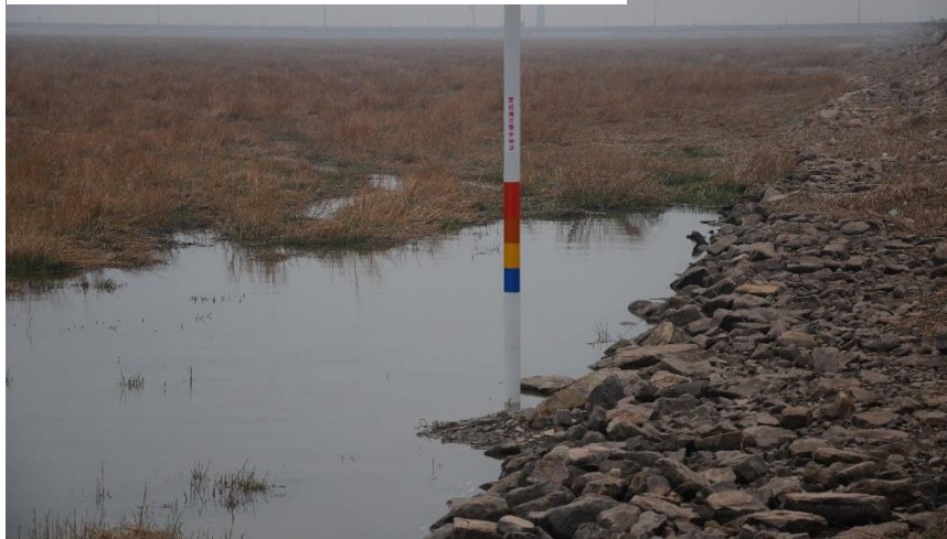
Warning water level gauge
